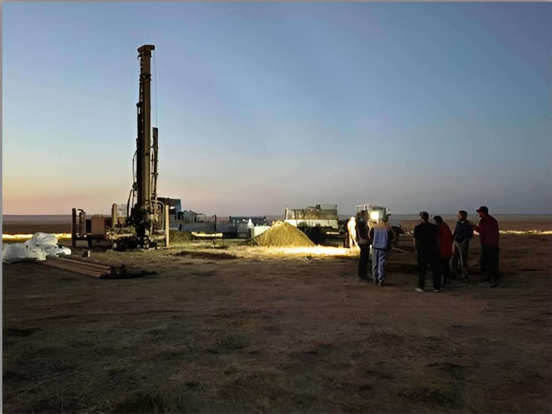
Waterwell rig at UNWH-01, Urgakh Naran
