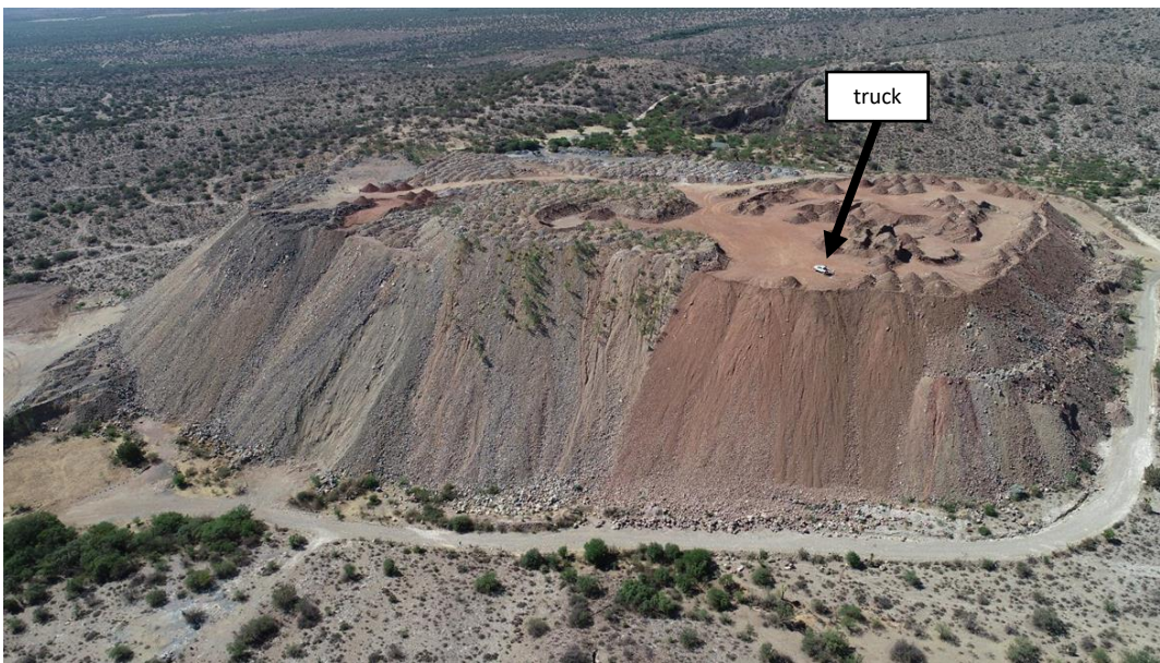
Open Pit Oxide Stockpile
